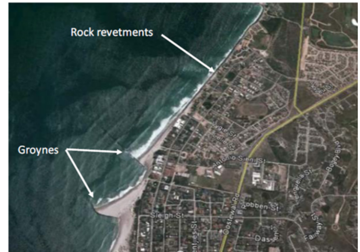
Figure 7: Groynes and rock revetment at Langebaan North beach Source: Saldanha Bay Water Quality Forum Trust 17
